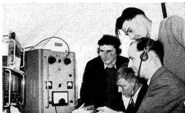
At G3EBH/P, one of the Lincoln stations, a modified LG300 transmitter was used with an 832 running 10 watts input in the p.a. (Photo by Lincolnshire Echo).
