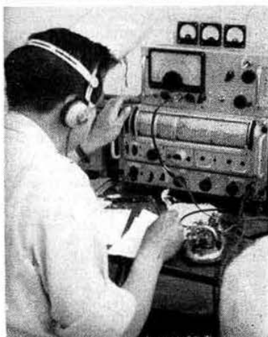
G3LOV trying to push the score above 200 contacts at Mitcham Group's G3JJG/P during the last few minutes of N.F.D.1958. The receiver is an ex-R.A.F. R1475.
